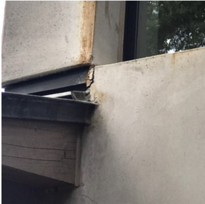
SIDING CRACK NEAR ROOF TRIM - RIGHT
