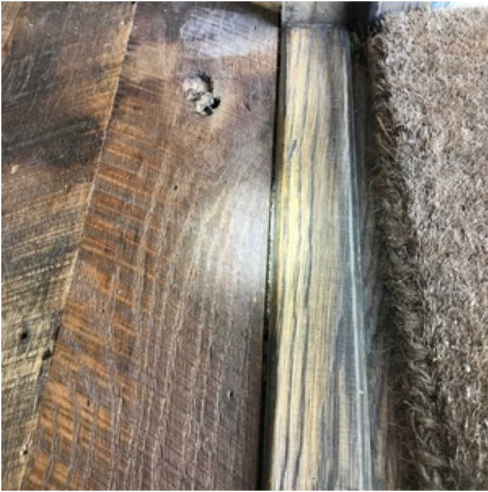
SEAL GAP - FRONT DOOR TRANSITION
