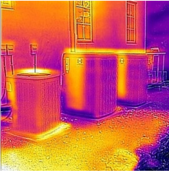
NORMAL READINGS - THERMAL CAMERA
