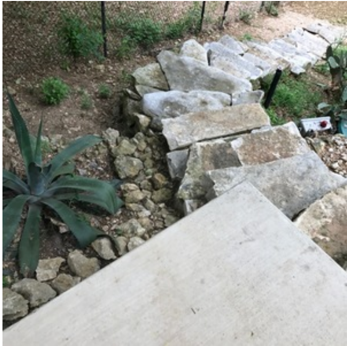
MISSING RAILING/UNEVEN STONE STEPS
