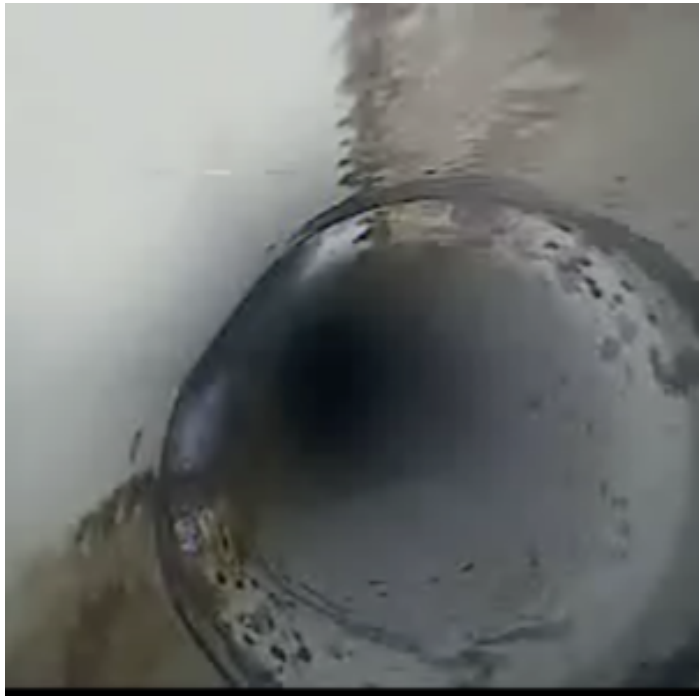
PIPE CAMERA - NO ISSUES OBSERVED
