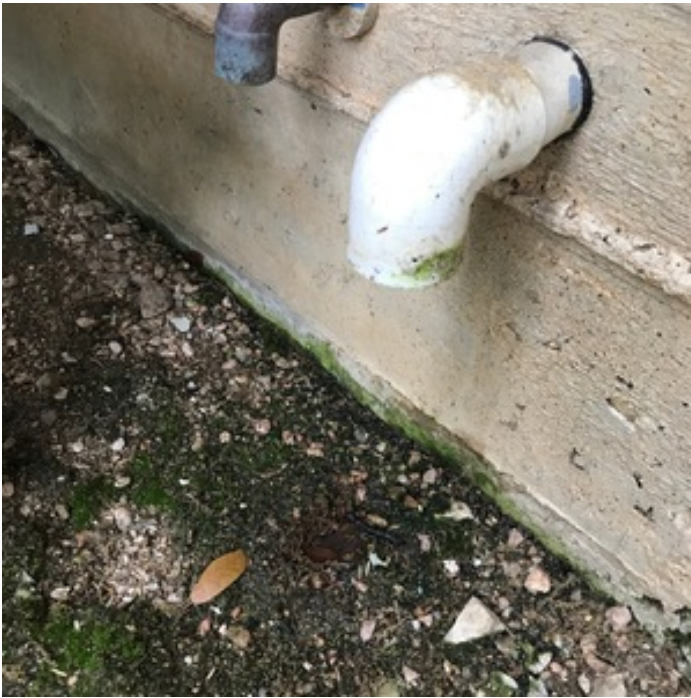
EXTEND CONDENSATE DRAINS
