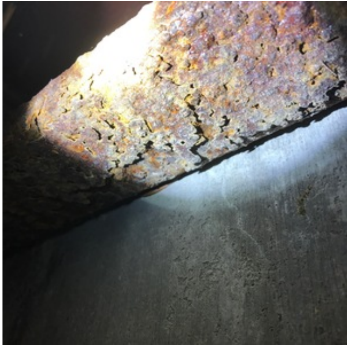
BEAM DAMAGE - POOL DECK
