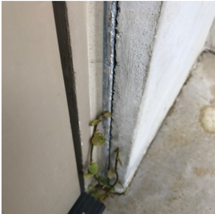
MINOR GAPS NEAR DOOR CONNECTIONS
