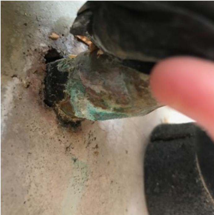
SUPPLY PIPE CORROSION
