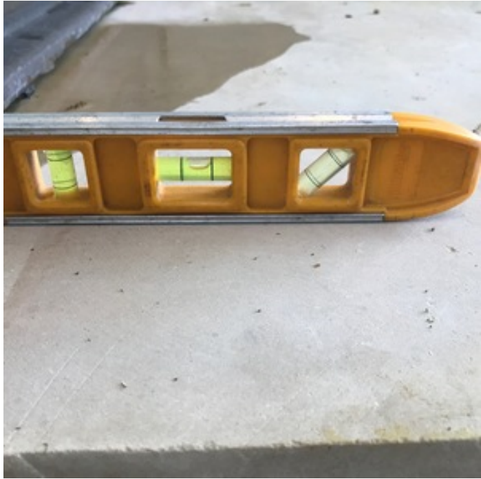
SLOPE CONCERN AT DOOR PAVERS
