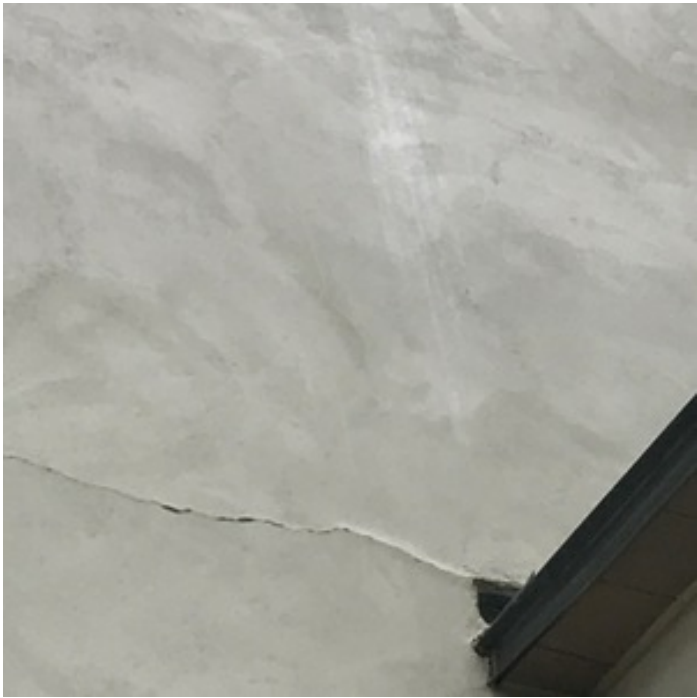
EXPANSION CRACKS/MOISTURE CASCADE
