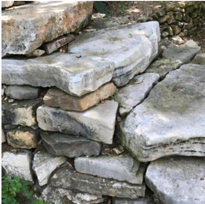
NO RAILING/DRY STACK STEPS
