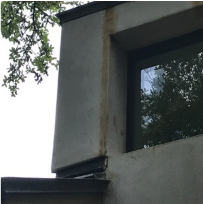
MOISTURE WICK NEAR FLASHING CRACKS
