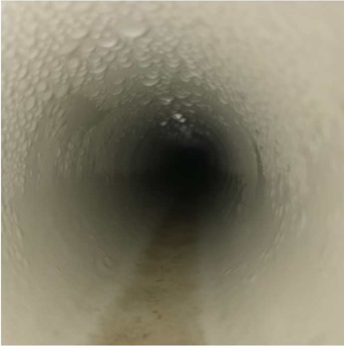
EXCESS CONDENSATE POOLING
