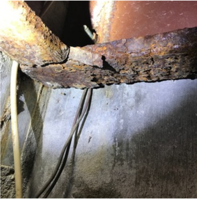
BEAM DAMAGE - POOL DECK
