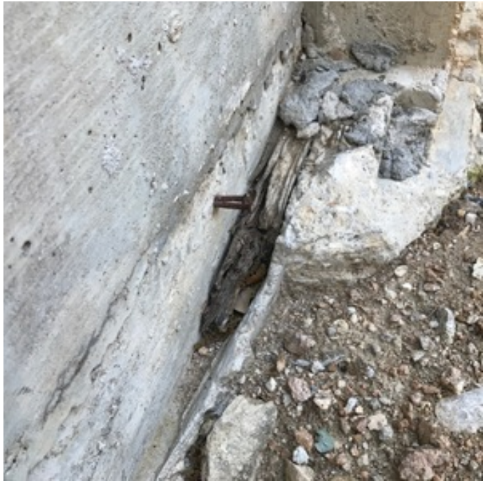
REMOVE FORM BOARD DEBRIS
