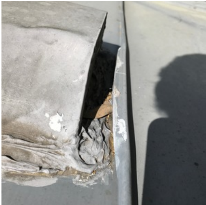
BOOT/SEAM CONCERN - LEFT SLOPE
