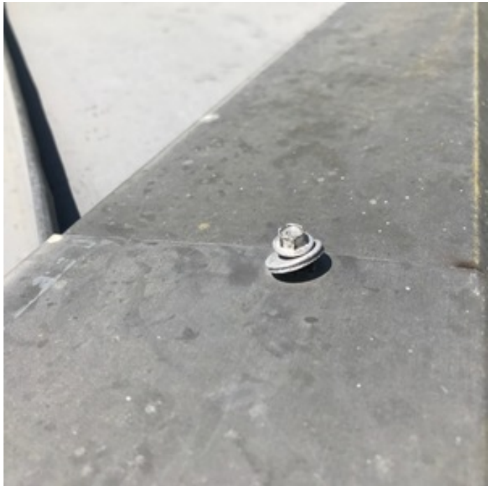
LOOSE SELF-TAPPING SCREWS
