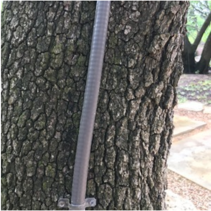
PROPER EXTERIOR WIRE PROTECTION
