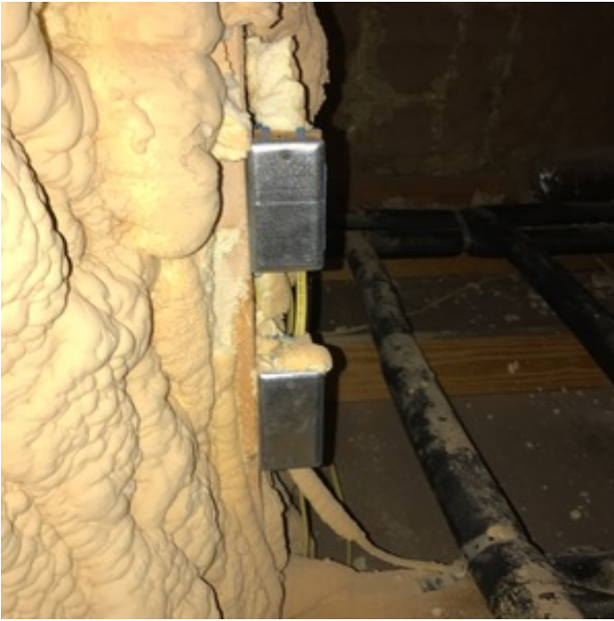
PROPER WIRE PROTECTION
