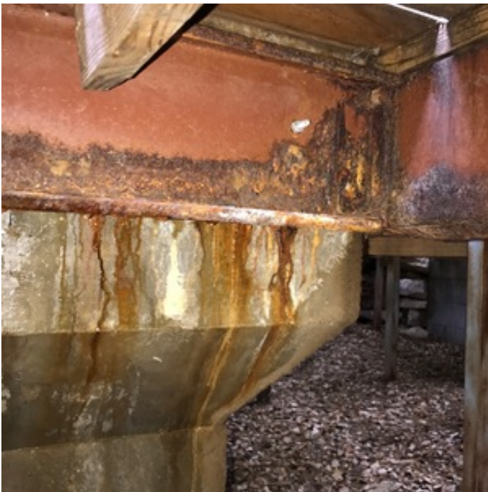
POOL LEAK/BEAM DAMAGE
