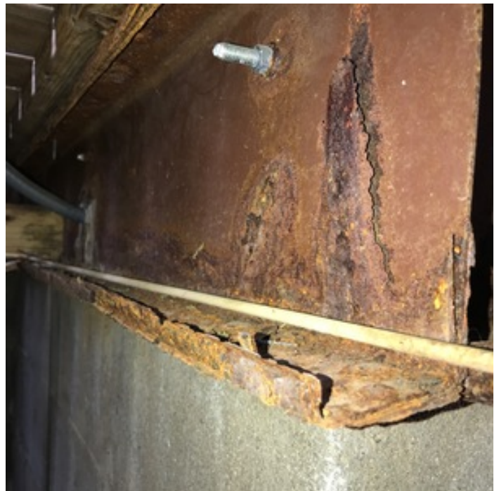
BEAM DAMAGE - POOL DECK
