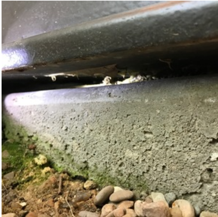
MOISTURE ENTRY - PAVER/THRESHOLD
