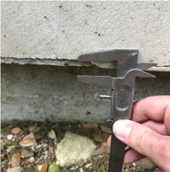
MATERIAL SEPARATION AT EDGE TRIM
