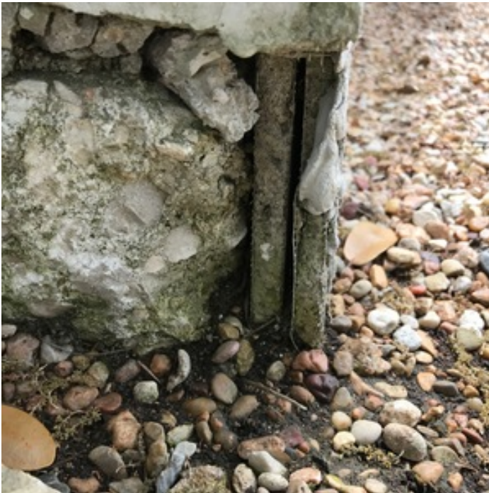
BACKER BOARD AT EXTERIOR WALL
