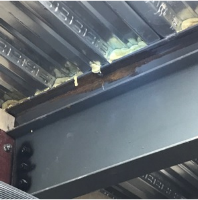
ISOLATED RUST AT I-BEAM
