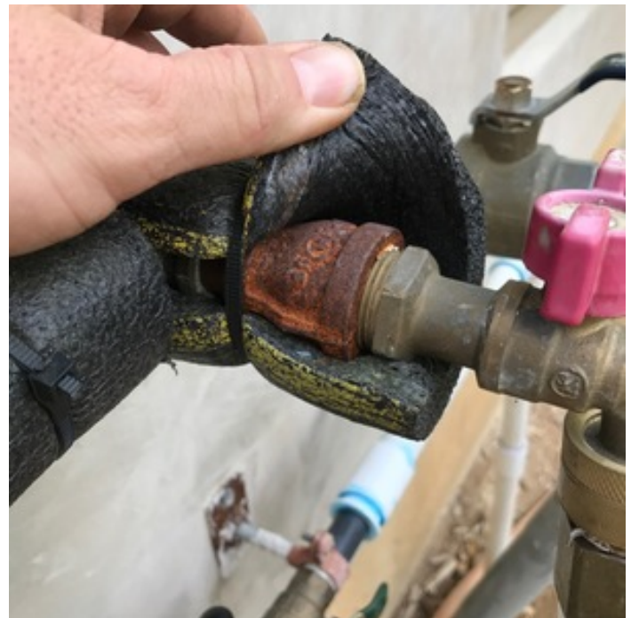
MINOR CORROSION AT BRASS/STEEL CONNECTION
