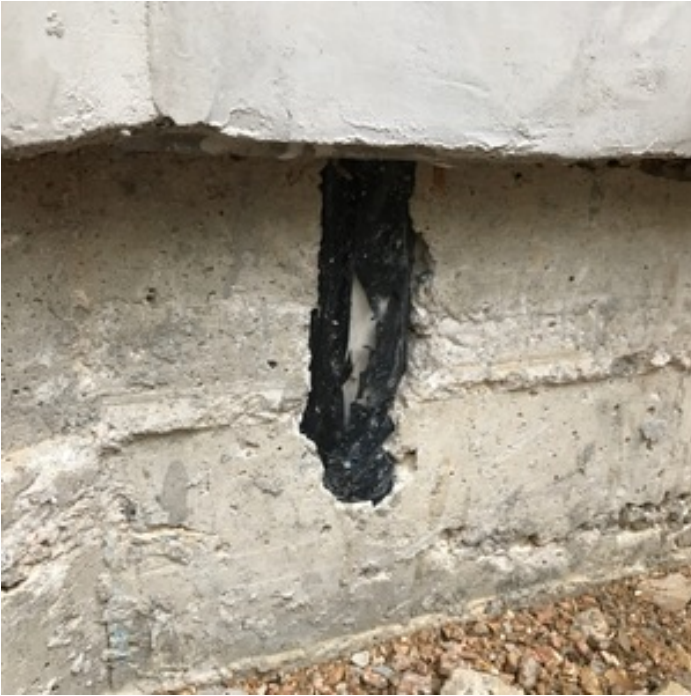
COVER/SEAL EXPOSED PIPE
