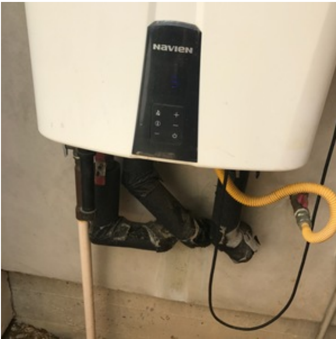
EXTEND CONDENSATE DRAINS
