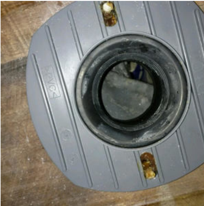
COMMODE DRAIN REDUCED (OVER 50%)
