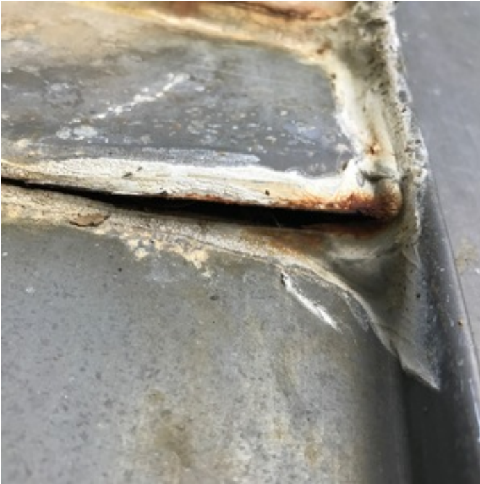
FLASHING/PANEL ISSUES - RIGHT SIDE
