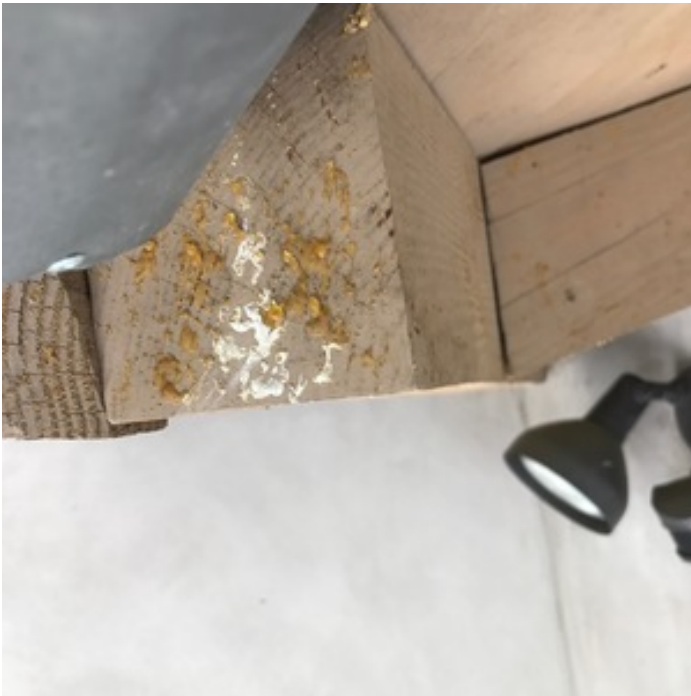
SAP/ADHESIVE AT SOFFIT FEATURES
