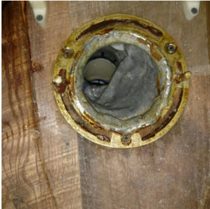
COMMODE DRAIN REDUCED (OVER 50%)
