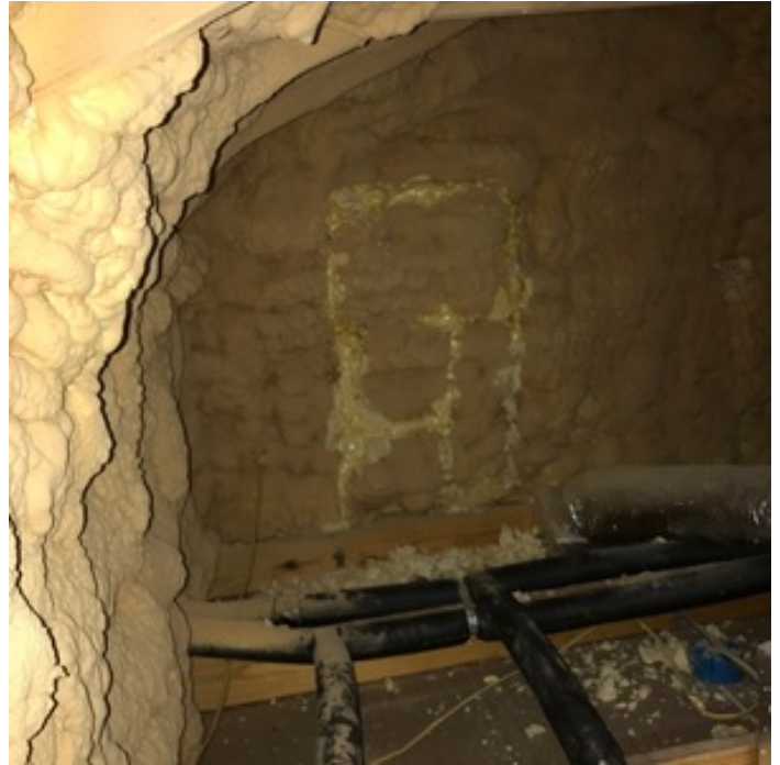
FOAM INSULATION AND PATCH
