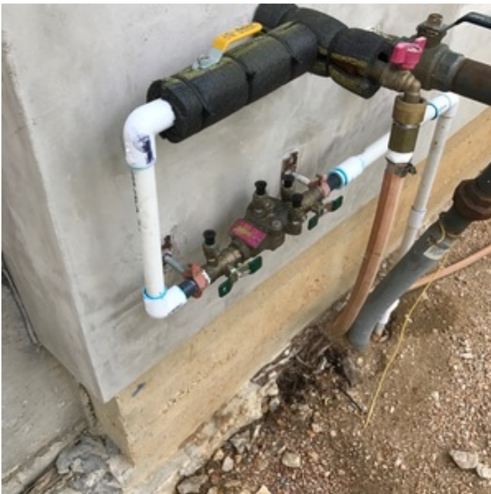
PROTECT/INSULATED EXPOSED PIPING
