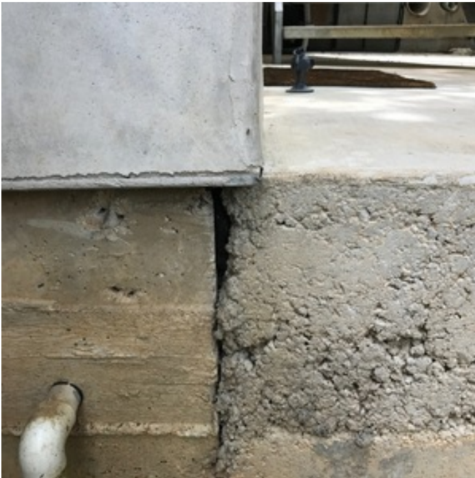
SLAB FLUSH WITH WALL
