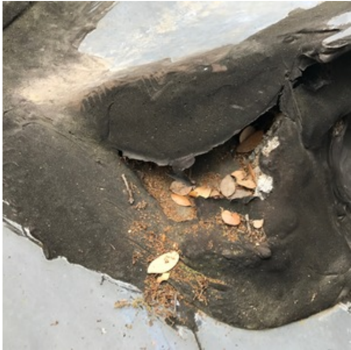
INSTALL/MOISTURE PENETRATION CONCERNS
