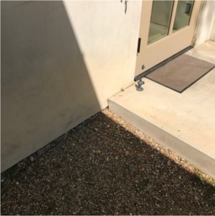
EXTERIOR FEATURES COVER FOUNDATION
