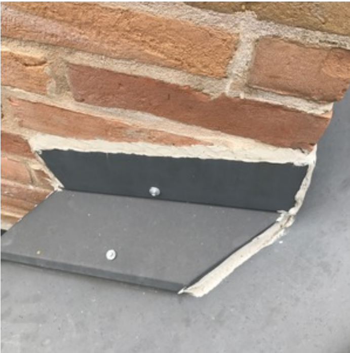
FLASHING INSTALL CONCERNS
