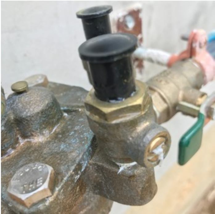
ACTIVE LEAK - PRESSURE VALVE
