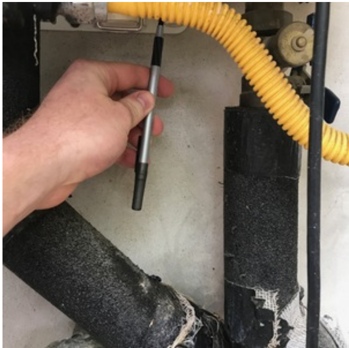
EXTEND CONDENSATE DRAINS
