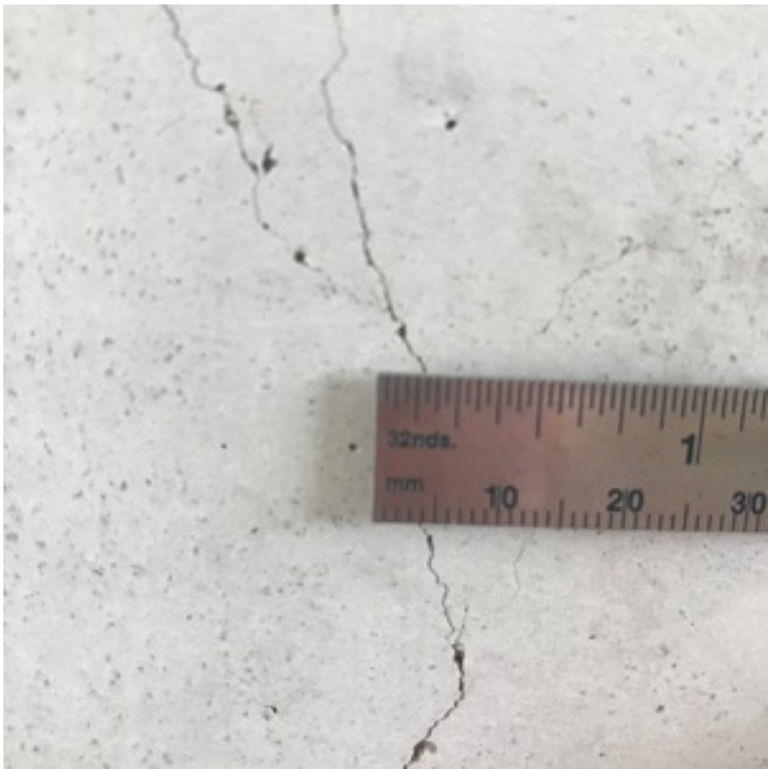
MONITOR NORMAL CRACKING
