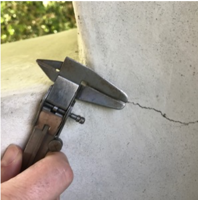
MONITOR NORMAL CRACKING
