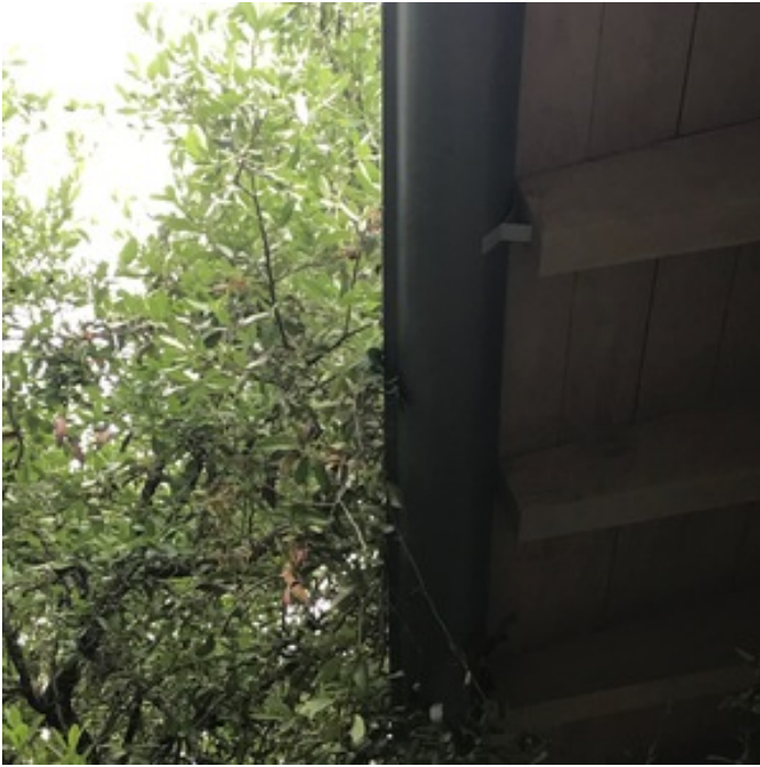
TREES IN CONTACT WITH GUTTERS/ROOF
