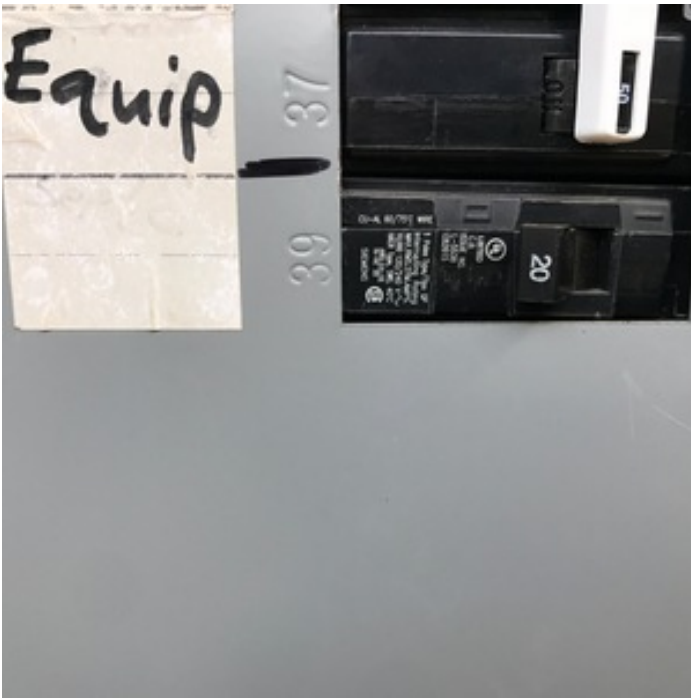
FAILED BREAKER - SEWER PUMP
