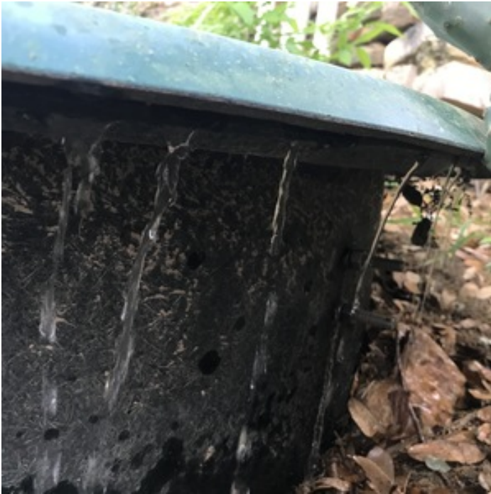
NON FUNCTIONAL/SUMP TANK OVERFLOW
