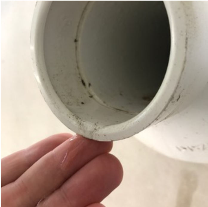
EXCESS CONDENSATE/EXHAUST FLUE
