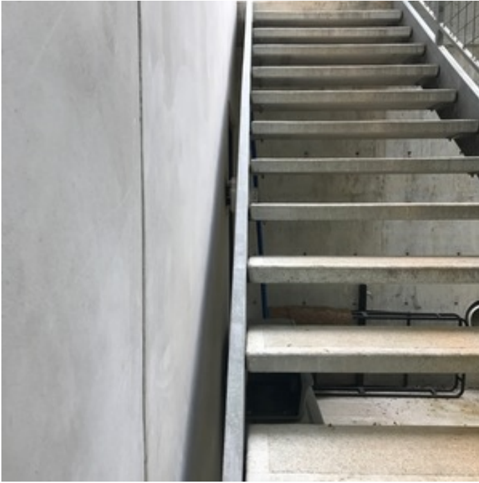
MINIMAL STRINGER BRACING/SUPPORT
