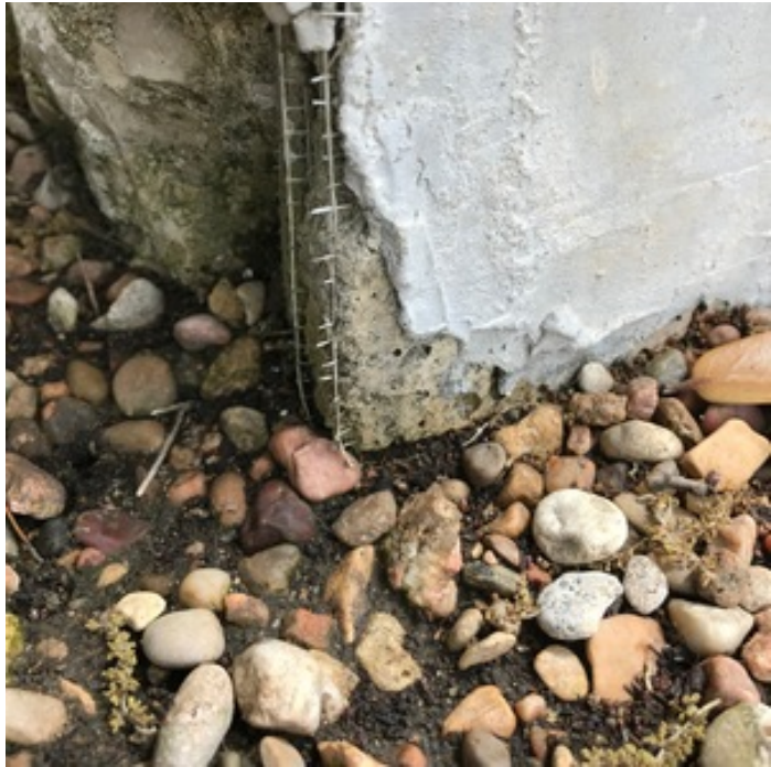
BACKER BOARD AT EXTERIOR WALL
