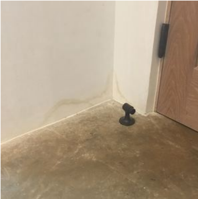
MOISTURE DAMAGE - KITCHEN AREA WALL
