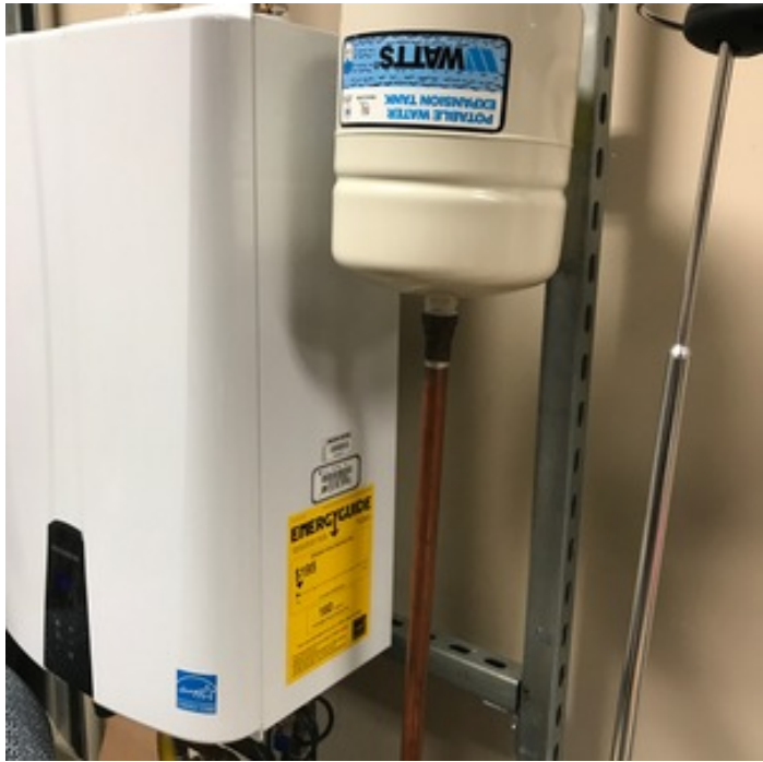
SECURE/LEAK PROTECT EXPANSION TANK
