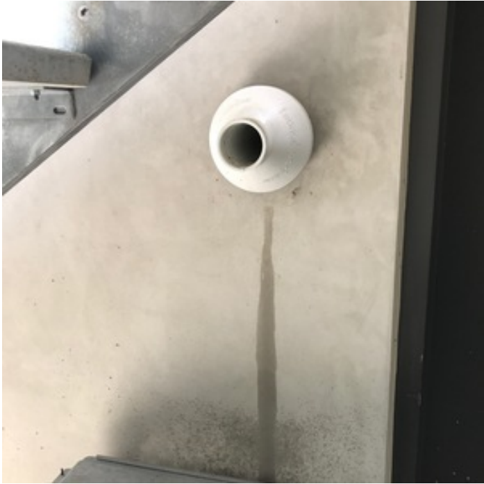
EXCESS EXHAUST MOISTURE
