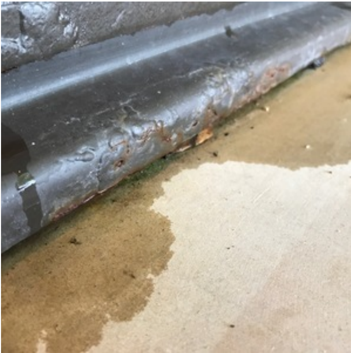
RUST/DAMAGE AT THRESHOLD
