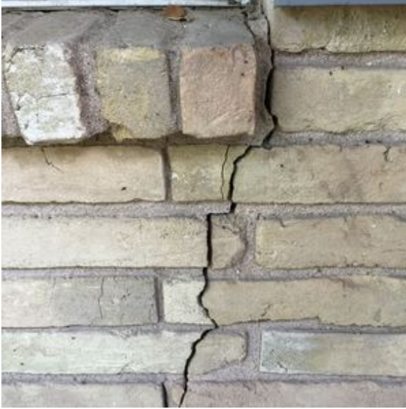
SETTLEMENT CRACKS - MONITOR
