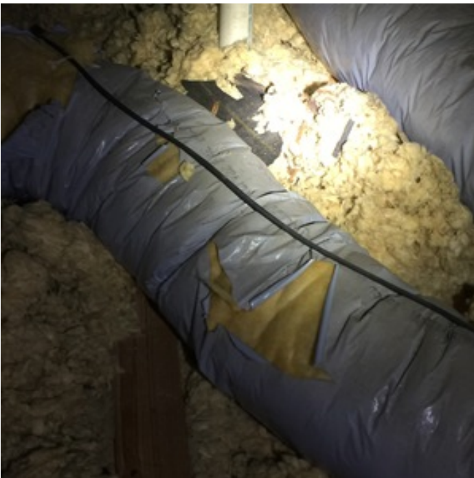
MINOR DUCT DETERIORATION
