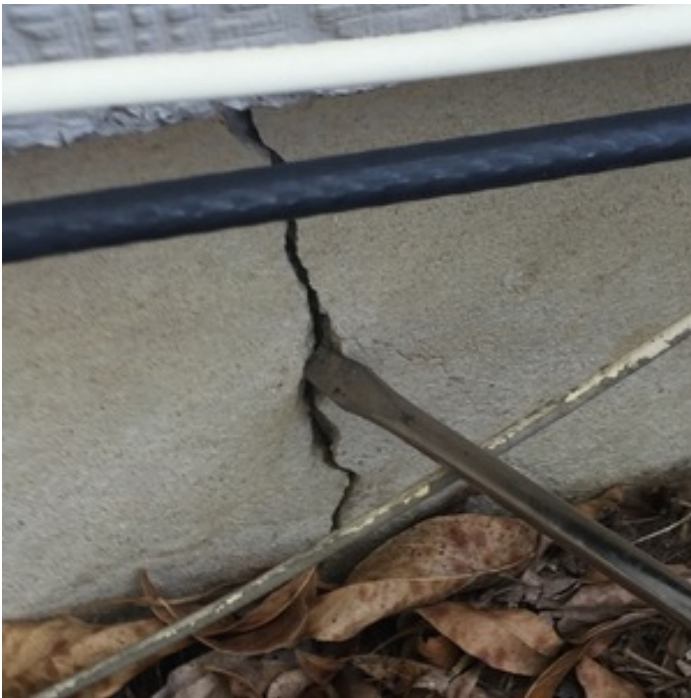
1/8" CRACK RIGHT FOUNDATION
