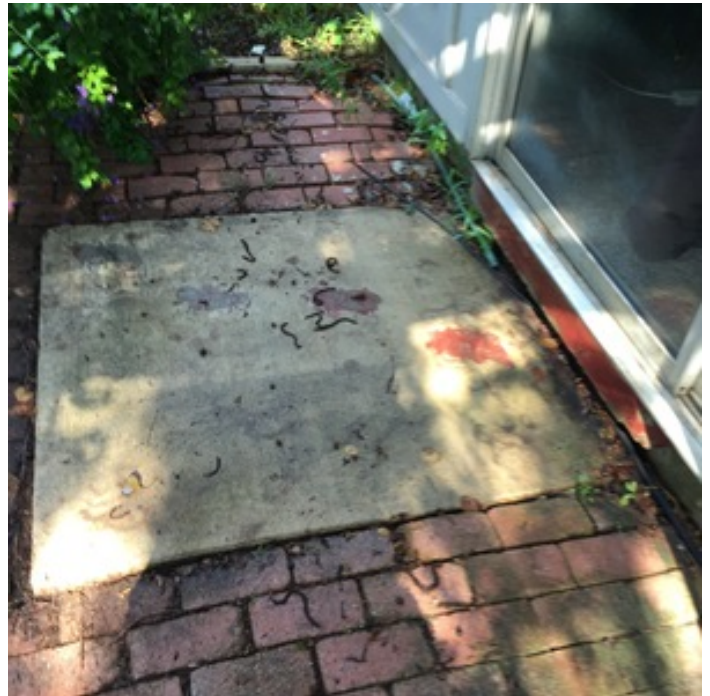
IMPROPER SLOPE AT BACK PORCH
