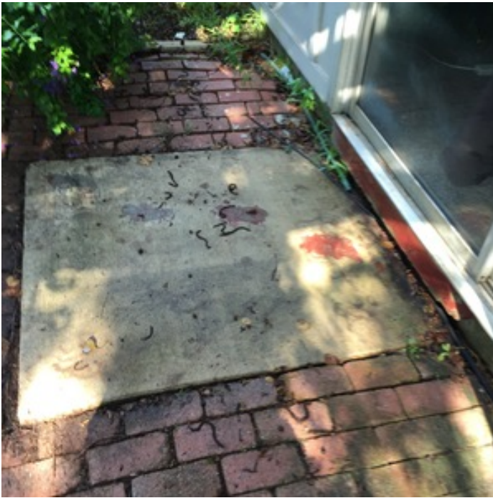
IMPROPER SLOPE BACK SLAB
