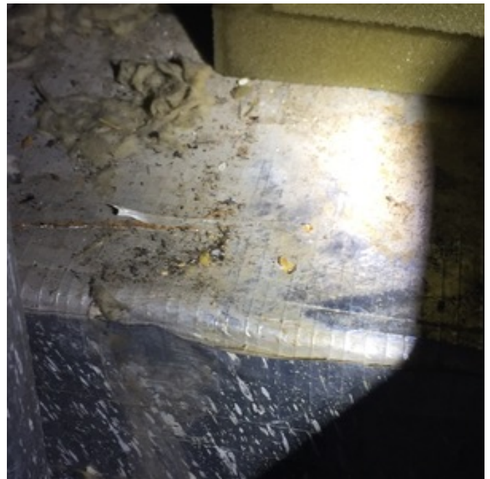
AIR GAP AT PLENUM
