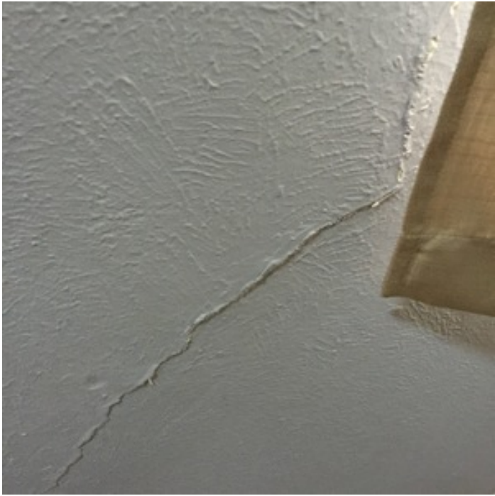
DIAGONAL WALL CRACKS
