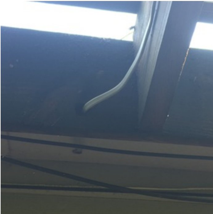
IMPROPER ELECTRICAL (EXPOSED WIRE)
