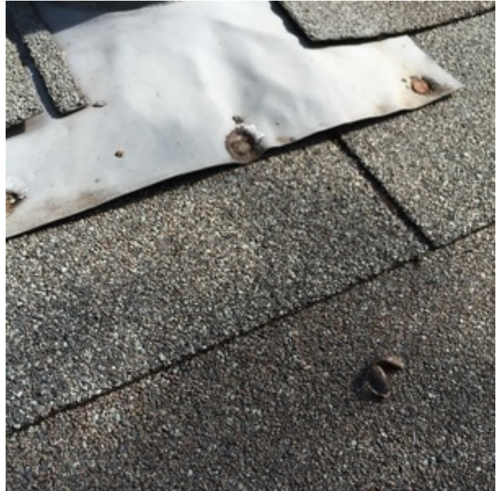
CAULK/SEAL NAIL HEADS
