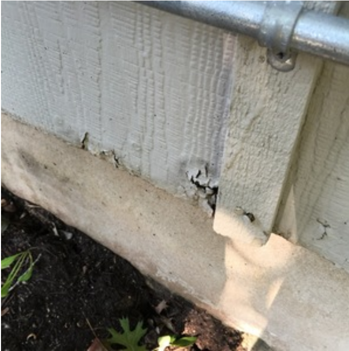
MASONITE DAMAGE
