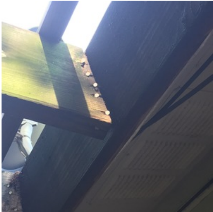
LOOSE/IMPROPERLY SUPPORTED FRAMING
