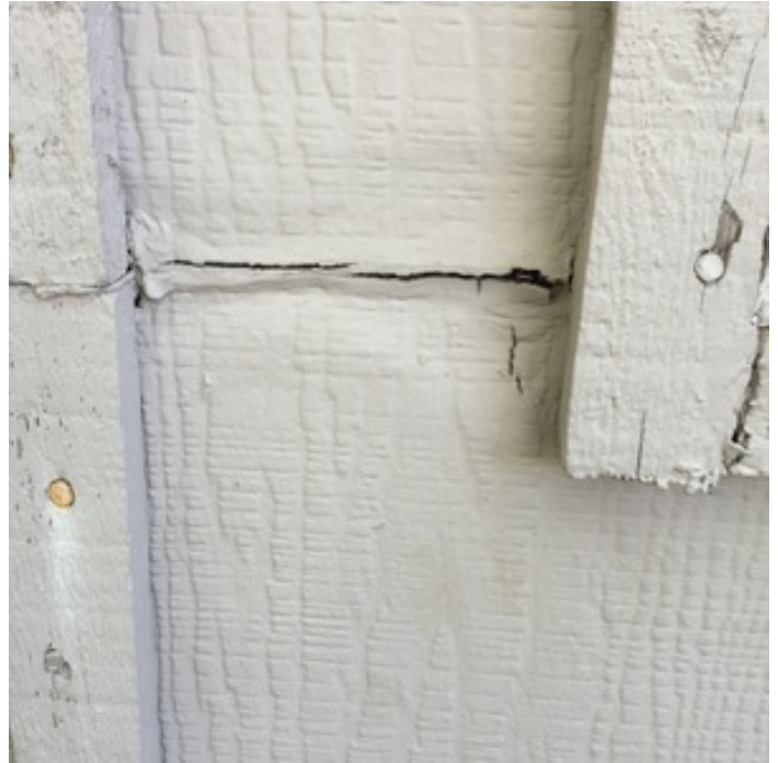
MASONITE DAMAGE
