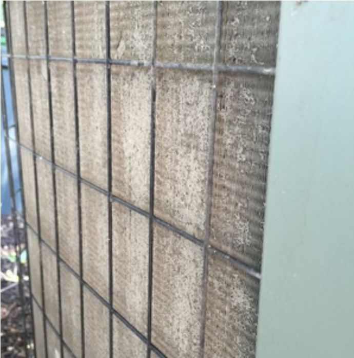
BLOCKAGE AT COIL FINS
