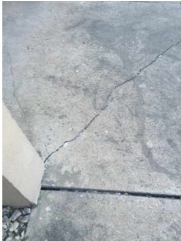
MINOR SETTLEMENT CRACK AT WALKWAY -NORMAL SETTLEMENT ONLY
