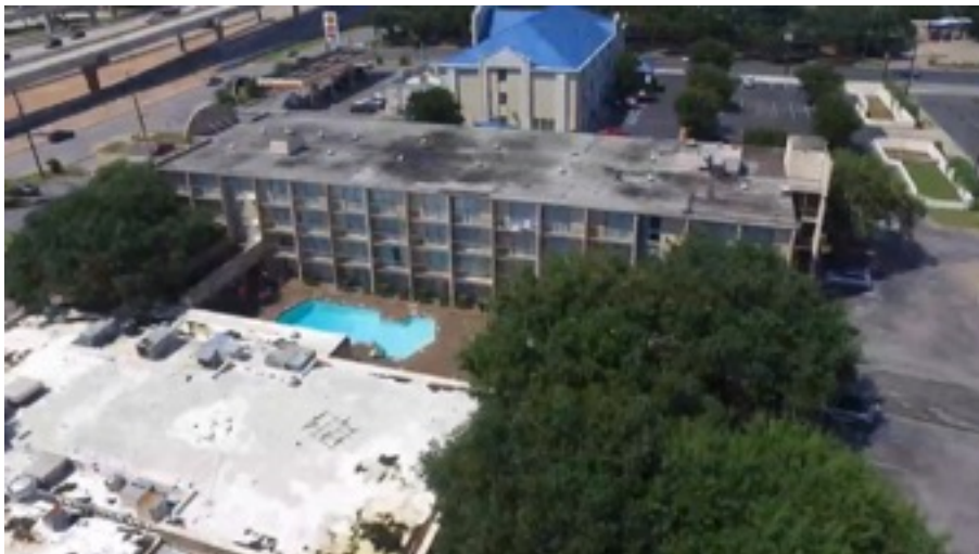
NO MAJOR STRUCTURAL ISSUES NOTED DURING DRONE ASSESSMENT (POOLING AT ROOF)
